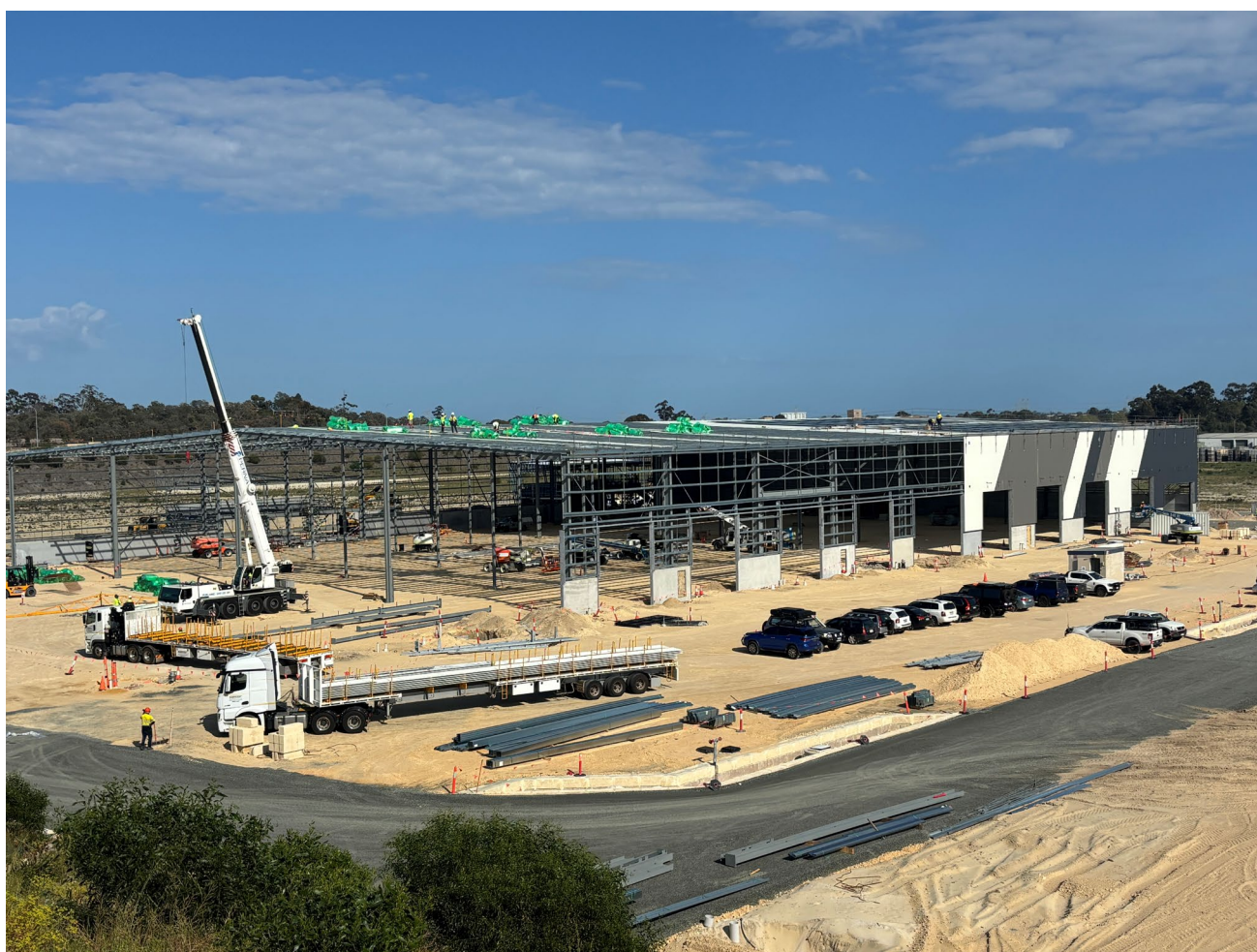
Image: First warehouse under construction.
