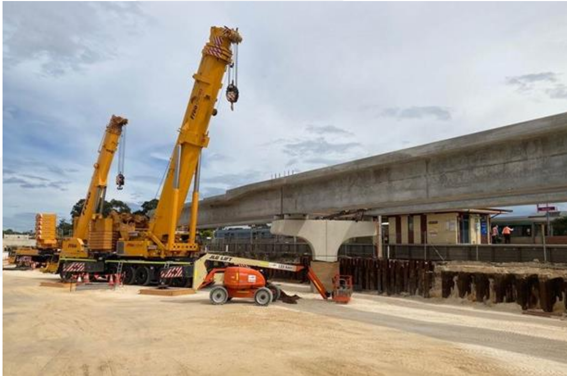
Beam Installations at Bayswater Train Station
