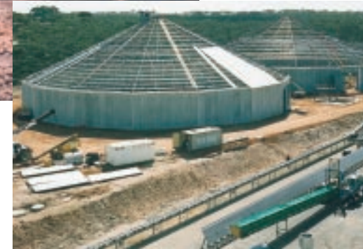
Bulkwest 20,000 tonne Grain Storage Cells.
