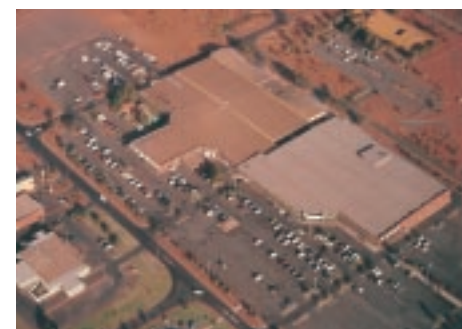
SOUTH HEDLAND SHOPPING CENTRE. (South Hedland, WA). Interest - 18.75%.
