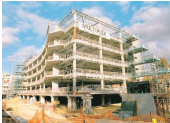
Ord Street Offices, West Perth.
