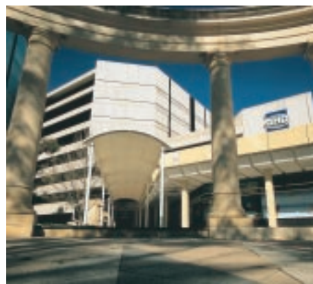
GHD HOUSE. (Adelaide Tce, Perth). Interest - 18%.
