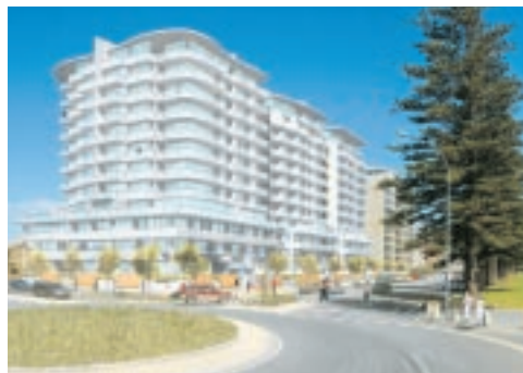
Liberty Towers, South Australia.
