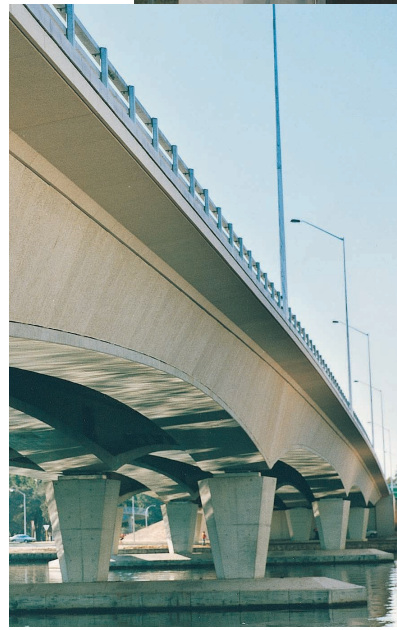
Narrows Bridge duplication - Perth.
