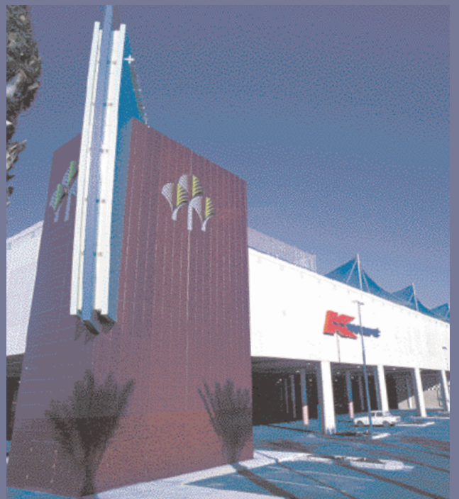
GARDEN CITY SHOPPING CENTRE. Special patterned wall panels painted to the clients' requirements.
