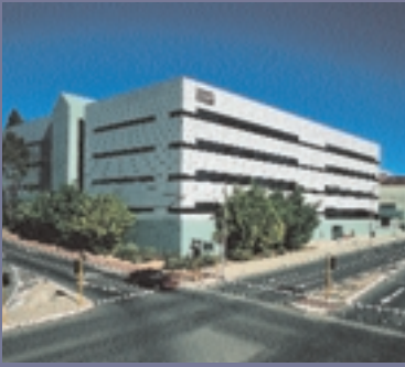
THE IBM CENTRE (Hay St, West Perth). Schaffer has a 22.1% interest in this property.
